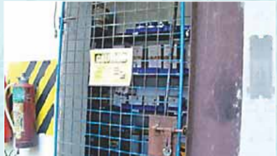
Chemical Storage Area- Caution Signage, Fire Extinguisher Nearby
